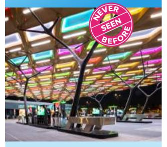
The UAE's national tree is renowned for its resilience to harsh weather conditions. The Service Station of the Future is built on an exoskeleton based on the ghaf tree structure, supporting a cutting-edge, solar-powered, carbon-fibre canopy.
